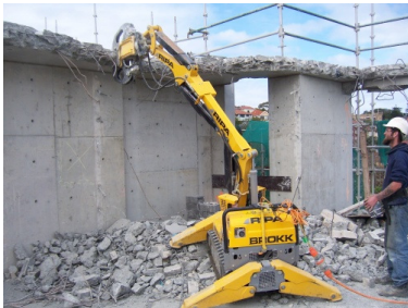
Photo from Brokk Website
