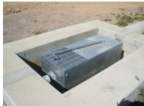
In the event of a major spill/emergency, the ball valve can be closed between the third chamber and the storm water outlet, thus eliminating external contamination.
