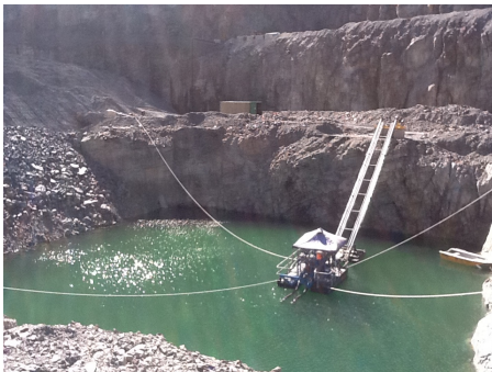
Newly Installed Floating Pontoon and Pump Lines
