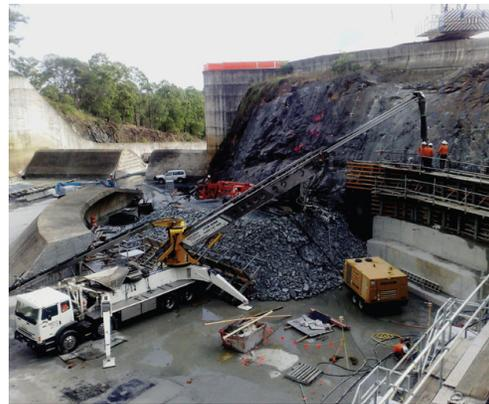
Example of road truck mounted mobile conveyor
